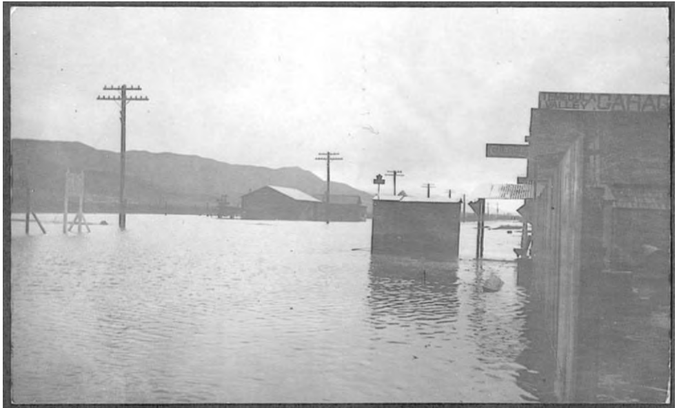
Looking north, the Murrieta Creek flooded Front Street in Temecula. The Temecula Valley Garage is on the right. Source: The Fernald Family Collection
