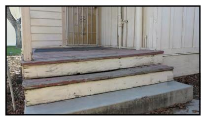
The wood on the museum's back porch was water damaged and deteriorating. The volunteers removed the wood and replaced it with a synthetic material that looks like wood, but is durable and will last for many years to come. They not only volunteered their time in making the repairs, but they also purchased and donated the materials. Thank you.
